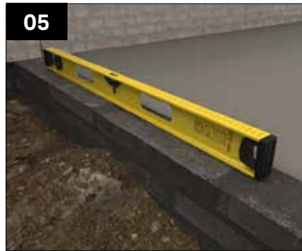
05 Ensure base is level. If required level off with metal or slate shims or a bed of mortar.
