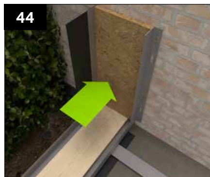
At the host wall, position the host wall tray onto the base tray below. Ensure the vertical DPC (step 8) is located into the brickwork and extends beyond the tray steel, this will need to reach the wall once angled away for access.
