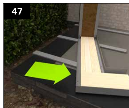
The base tray can now be angled away from the boundary by sliding on the skids to enable access. The hinged steel should bend along the perforations, whilst stabilising the wall.
