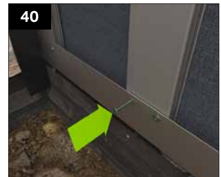
Secure the base trays through the two pre-punched holes into each of the walling panels/clips using the GPHS fixing provided.
