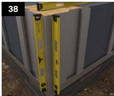
Ensure that the building is plumb and level.
