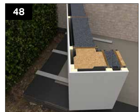
This section of wall can then be constructed following the standard process shown from step 23, it may be advisable to fit the roof eaves beam whilst external access is available. Once the wall has been cladded externally with membrane, battens and calcium silicate board and any final wall finishing it can then be moved into its final position. See page 29 for fitting battens and calcium silicate board.
