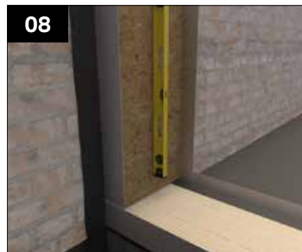
08 The host wall tray can be used to strike a plumb datum line down from the host wall. This can then be used to find the correct position for the base trays.
