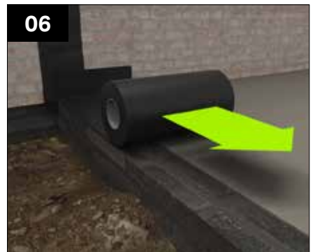
06 Position horizontal DPC (NOT SUPPLIED, 300mm min. recommended) around the perimeter of the base aligning with the external face and lapping up the host wall. Where walls are to be positioned, the DPC should run past the base trays, by minimum of 50mm, allowing for it to be lapped up the aperture face of walling.
