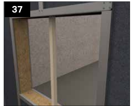
Leave the prop in place, this can be removed later once the clips are secure into the beam or tray above (roof dependant).
